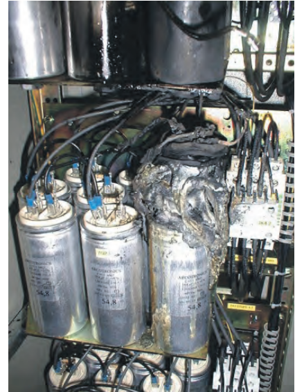
Fig.: Capacitors destroyed due to harmonics
